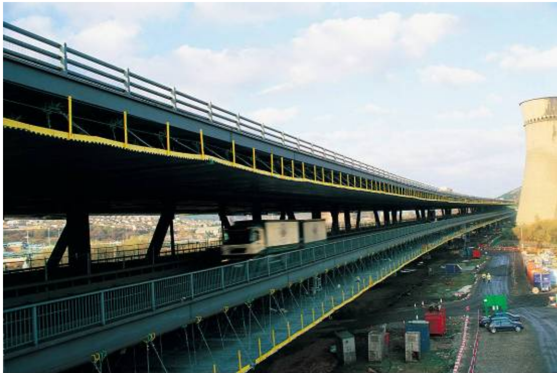
Two levels of Safespan 1 Kilometre long x 35 m wide on the Tinsley Viaduct in Sheffield
