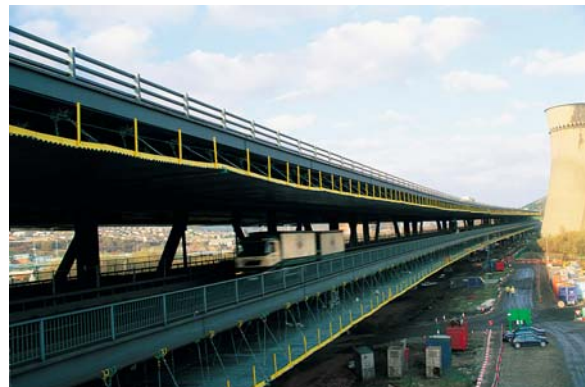
Two levels of Safespan 1 Kilometre long x 35 m wide on the Tinsley Viaduct in Sheffield
